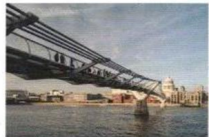
▲ Figure 3 The Millennium Bridge across the Thames, now with added dampers
