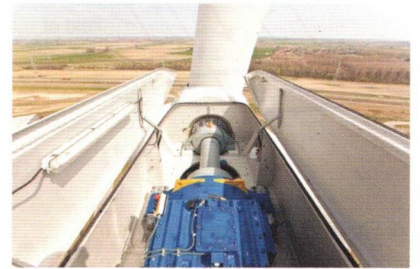
▲ Figure 1 The generator inside a wind turbine produces electrical energy by electromagnetic induction
